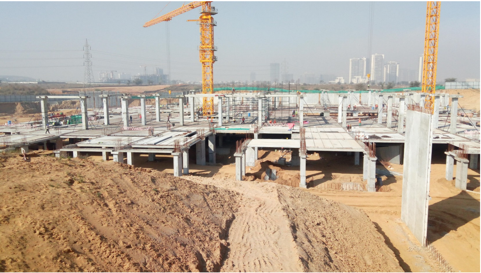
Isolators now under Installation
